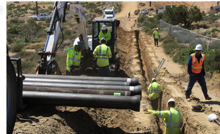
Camares Road Mainline Replacement
